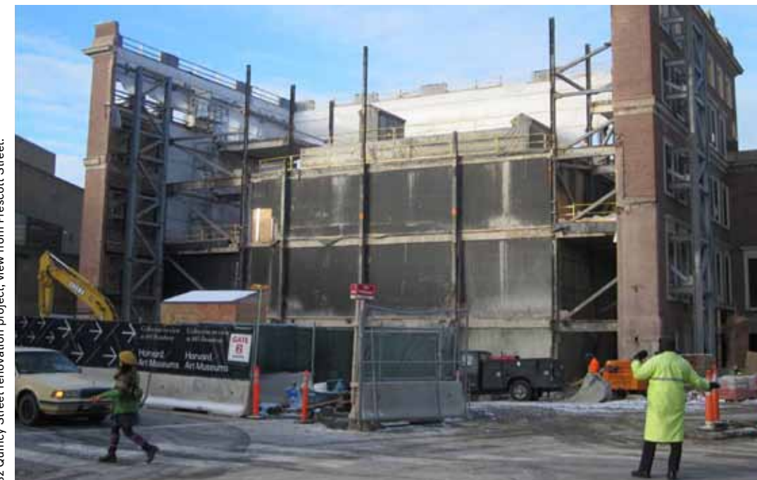
32 Quincy Street renovation project, view from Prescott Street.
